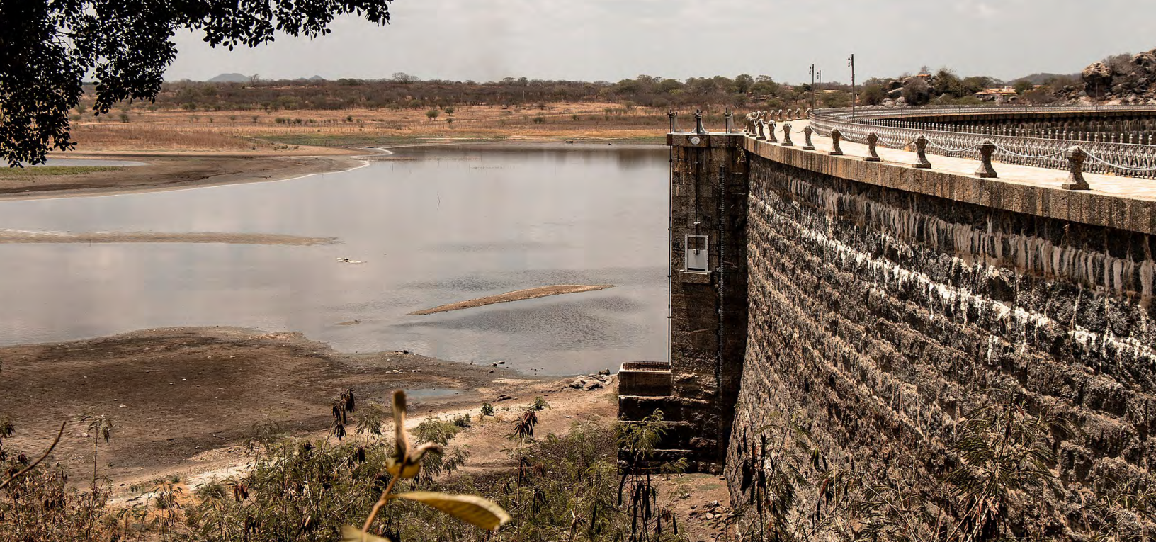
Exposed Water Height Marker and reservoir in dead volume during the 2016 Drought. Açude do Cedro, Quixadá - CE , Brasil. September 2016. EUCLIDES GABRIEL BRITO MEDEIROS
