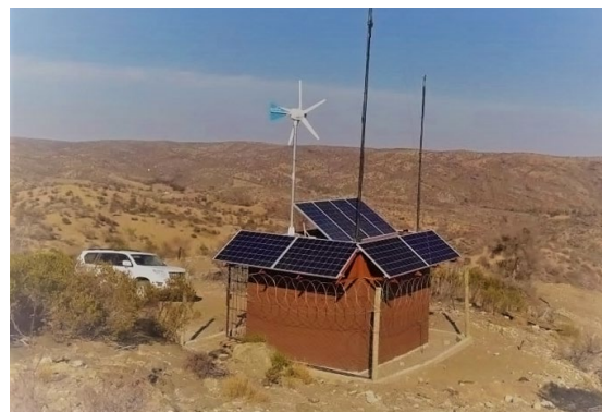
EMBASSY WINDHOEK'S SOLAR- AND WIND- POWERED RADIO REPEATER TOWER
